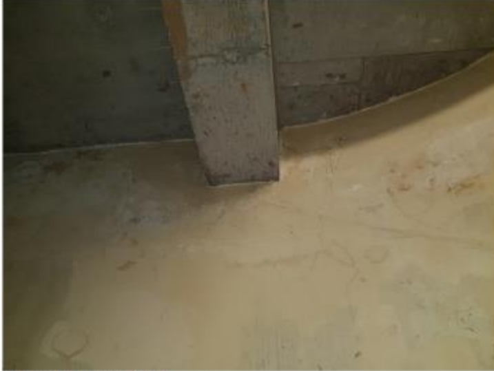
Figure 31: Damp Walls in Fire Escape
