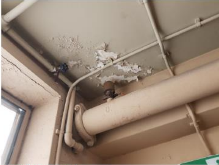
Figure 29: Spalling Concrete
