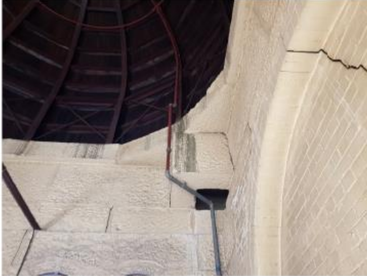
Figure 35: Water Staining From Dome Roof
