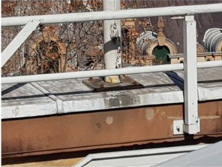
Figure 5: Corroded Flag Pole Connections South End
