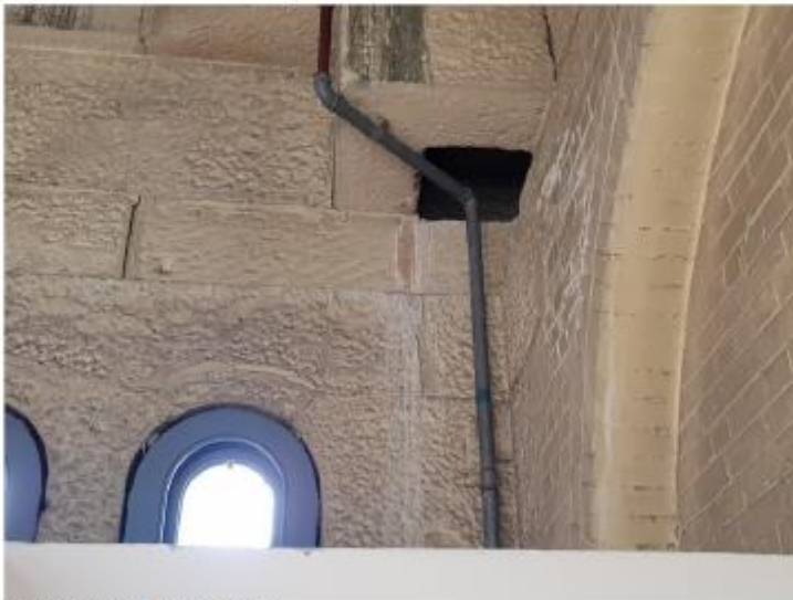
Figure 36: Water Staining From Dome Roof
