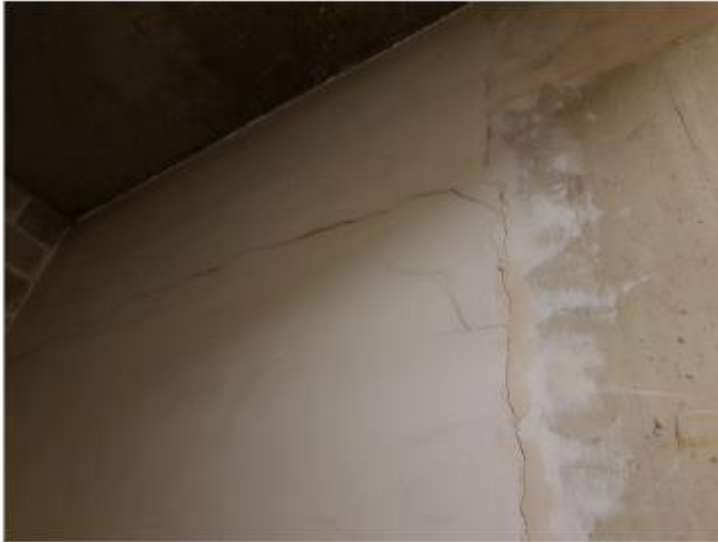
Figure 27: Fire Escape Cracking
