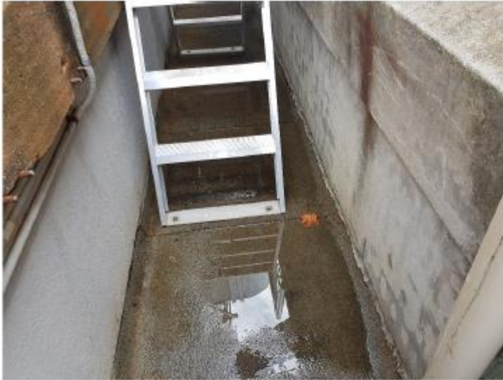
Figure 33: Ponding Water on North East Flat Roof
