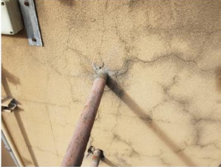
Figure 9: Cracking Around Embedded Railing
