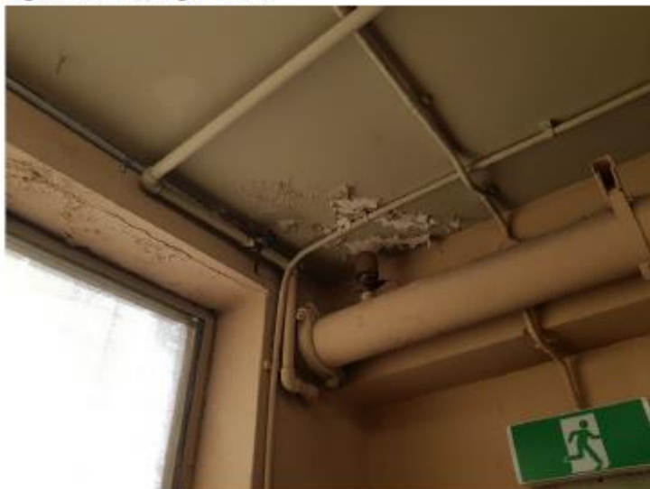
Figure 25: Cracking in Lintel
