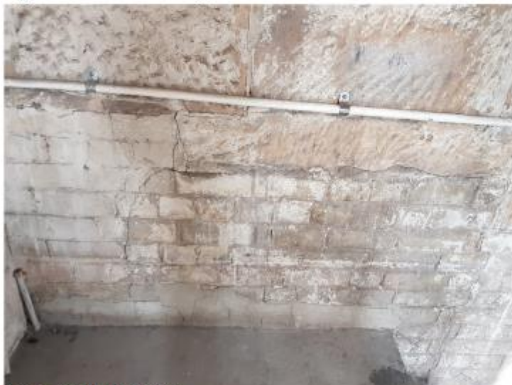
Figure 18: Vertical Cracking at Sandstone Brick Interface
