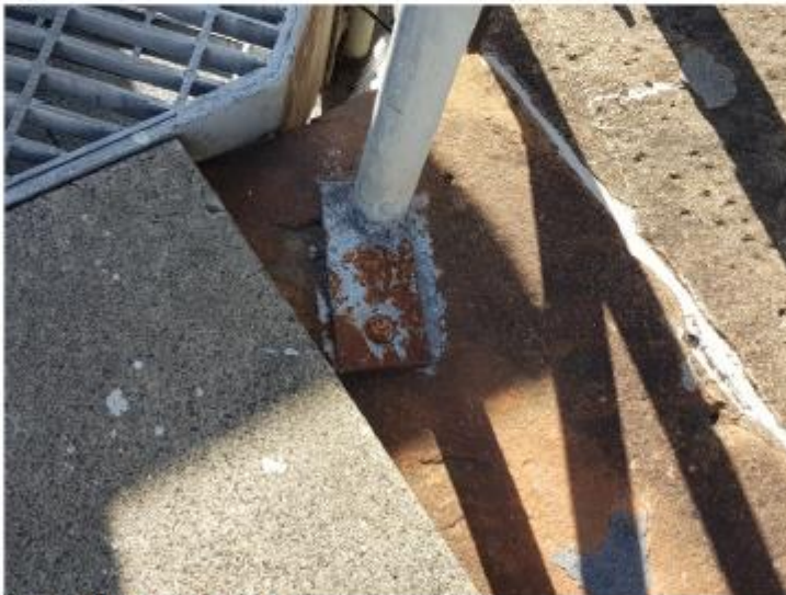
Figure 10: Corroded Connection of Access Structure South End
