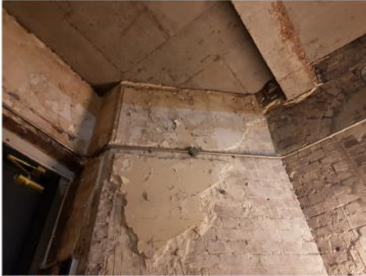
Figure 41: South Fire Escape Damp and Spalling Concrete
