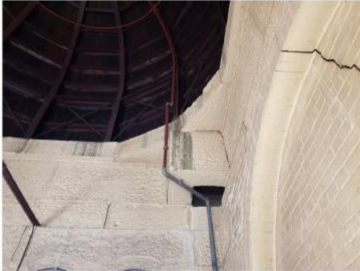
Figure 23: Vertical Cracking in Dome Masonry
