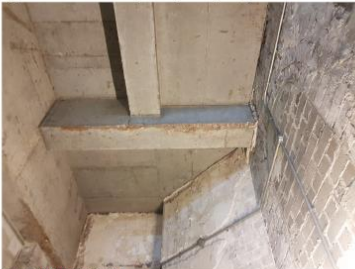
Figure 42: South Fire Escape Damp and Spalling Concrete
