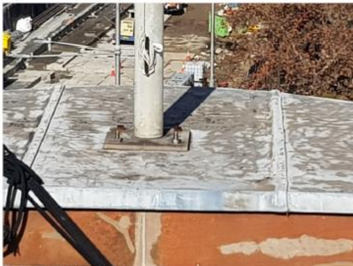
Figure 4: Corroded Flag Pole Connections South End
