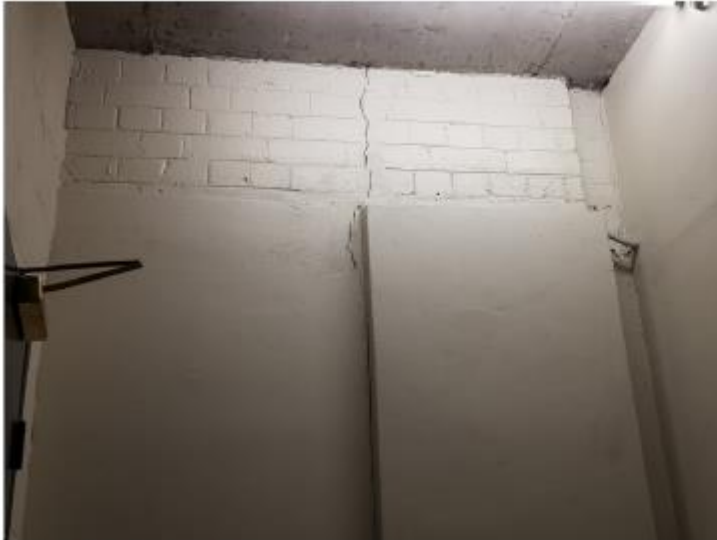
Figure 21: Vertical Cracking in Masonry
