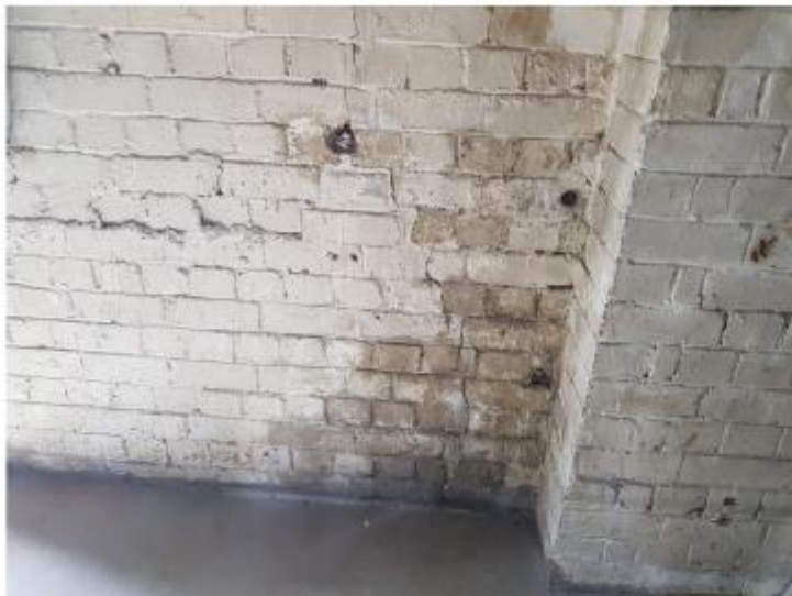
Figure 17: Cracking Around Old Embedded Fixings
