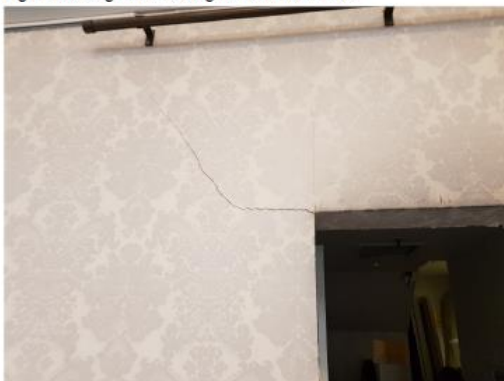
Figure 26: Diagonal Cracking in Tea Room Lintel
