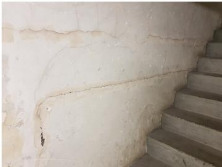
Figure 19: Cracking in Northern Fire Escape Walls
